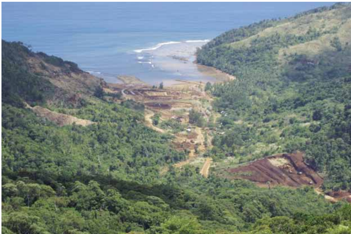
Aerial view of Acoje Operations.
