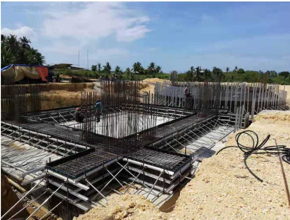
PREHEATER FOUNDATION AND RAW MATERIAL SILO FOUNDATION
