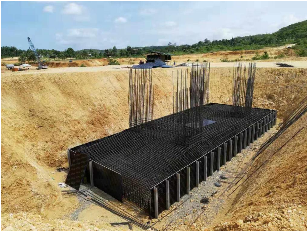
KILN 2 AND KILN 3 FOUNDATION
